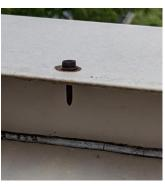
Leaks have been reported on the SSMR in several places. Other than chalking of the painted finish, the SSMR surfaces appear to perform well. and all appear to be due to deteriorated sealant and fasteners.
