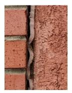
No specific exterior wall issues were reported regarding water infiltration; however, we did discover areas where sealant has failed and conditions where water runoff has stained the masonry below.
