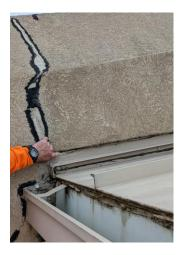
Surface cracks were found at various transitions where expansion occurs. Some cracks have been repaired with sealant; however, without a sufficient expansion joint to allow for both buildina thermal movement and contraction and expansion, the cracks will forever continue to worsen and fail allowing moisture to enter assembly. And without a way to vacate the system, deterioration of the EIFS will continue and eventually deteriorate.
